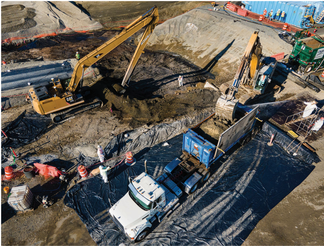
Excavator at right loads final bucket of chromium-impacted soil from sites south of Carteret Avenue.
