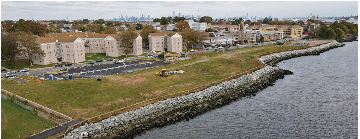
The remediation of a 5.2-acre portion of Dennis Collins Park includes a bigger and heavier rock revetment on the shores of the Kill Van Kull.
